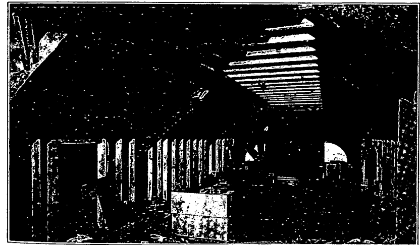
Illustrating Armstrong's Corkboard being applied on the underside of roof rafters in a residence.
