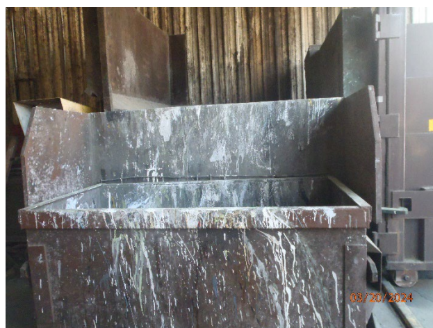
Picture 22 – Hazardous Waste Compactor
