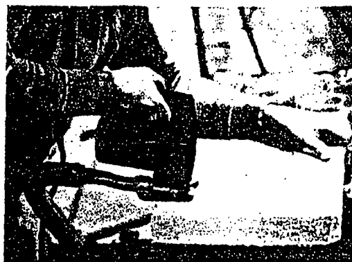
Right: A saw with a local ventilation system sucks up asbestos dust into a container. The OSHA standard specifies that hand or power-operated tools that produce asbestos dust must be equipped with local exhaust ventilation and dust collectors.
