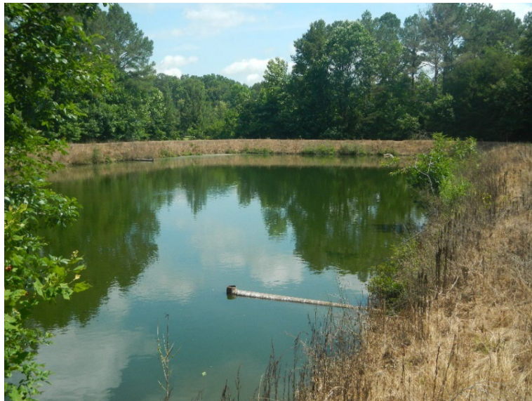
Figure 1. View of Grand Oaks wastewater treatment lagoon
