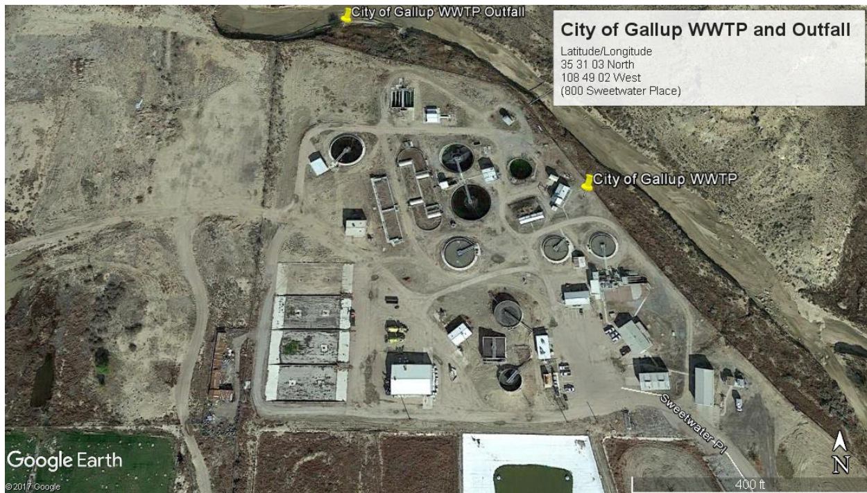
Image 1: Overall view of the City of Gallup's Wastewater Treatment Plant. Aerial from Google Earth maps.
