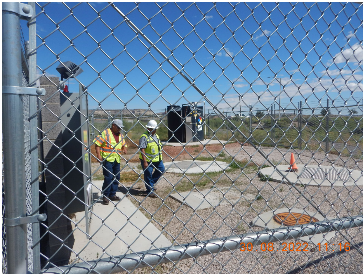
City of Gallup- Indian Hills Lift Station. Fenced enclosure. Lacking signage, does have stub-out for back-up power and audible alarms (DSCN2302). Photographed by D. Esparza
