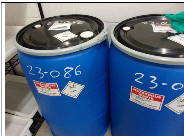
Figure 11: 9:50 AM Non-Flammable Organics Section (Photo 2 of 2) Two (2) 55-gallon containers with hazardous waste labels, accumulation start dates, and indication of the hazards of the contents.
