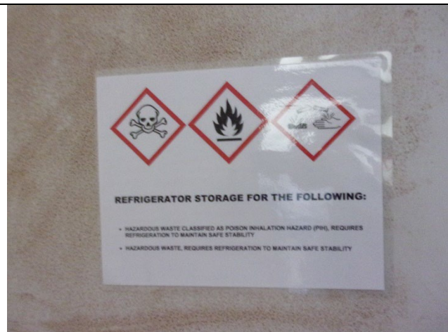
Figure 18: 9:58 AM Reactives Room Display label for blast-proof refrigerator.
