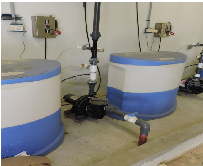
Picture 145 - UPR SWIMMING POOL AREA - At the Swimming Pool Area, all choline treatment at the swimming pool area is contracted out and is based on solid dosage of Sodium Chloride (NaCl) by a Pulsar 4 System .
