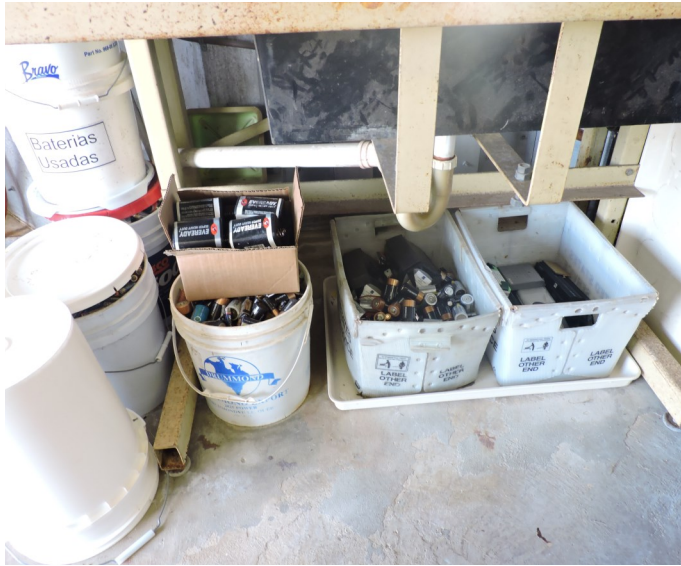
Picture 89 - UPR CENTRAL ACCUMULATION AREA- At the CAA, there two (2) plastic trays with discarded alkaline and computer lithium batteries, open and not clearly as “Hazardous Waste,” nor dated with their accumulation start dates and no hazard communication pictogram as, “Ignitable and Reactive Solids.”
