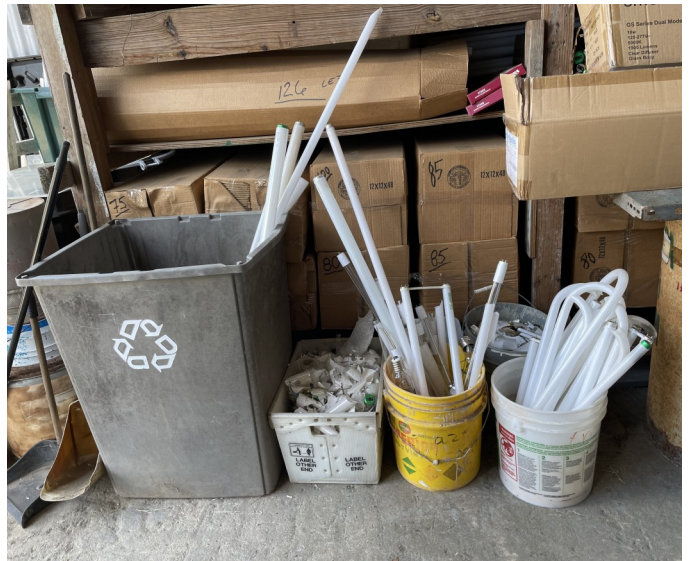
Picture 112 - UPR BUILDINGS & LAND DEPARTMENT - At the Universal Waste Storage Area there was one (1) white plastic tray (1'x1'x 2') with crushed fluorescent lamps and sodium bulbs showing evidence of breakage, leakage, and damage that caused releases of mercury or other hazardous constituents to the area.
