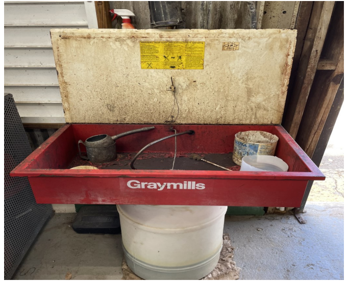
Picture 106 - UPR BUILDINGS & LAND DEPARTMENT- At the Fields and Roads Shop there was one (1) 30-gallon container part-washer machine which uses mineral spirit degreaser to clean up equipment parts served by Oil Energy System which was out of service for a long period of time.
