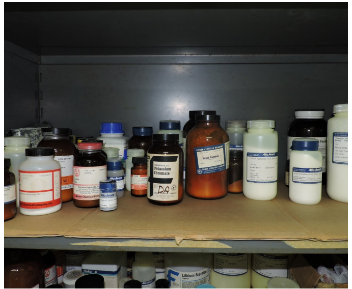
Picture 162 - UPR PHYSICS DEPARTMENT- At the Physics Lab F-129, there was potassium dichromate (oxidizers), stored next to Strontium hydroxides and lithium hydroxide (inorganic bases) incompatible and stored together without any mean of physical segregation nor hazardous waste determination
