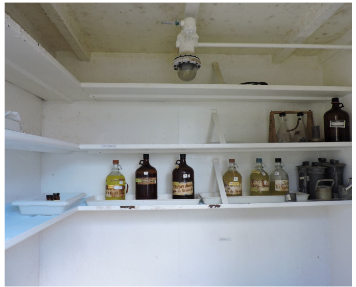
Picture 94 - UPR CENTRAL ACCUMULATION AREA- At the Hazmat Storage Building there were six (6) 1-gallon crystal containers with radioactive waste of "Uranyl Nitrate" and "Uranyl Acetate," stored for years without no hazardous waste determination or managed as hazardous waste (radioactive-corrosive).
