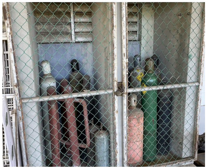
Picture 124 - BUILDINGS & LAND DEPARTMENT — At the Welding Shop, there were over ten (10) 100-lbs, 75-lbs and 25-lbs gas cylinders store in a concrete shed and secured with a cyclone fenced gates. There was oxygen, ethylene and other compressed gases stored in this shop and used for welding jobs.
