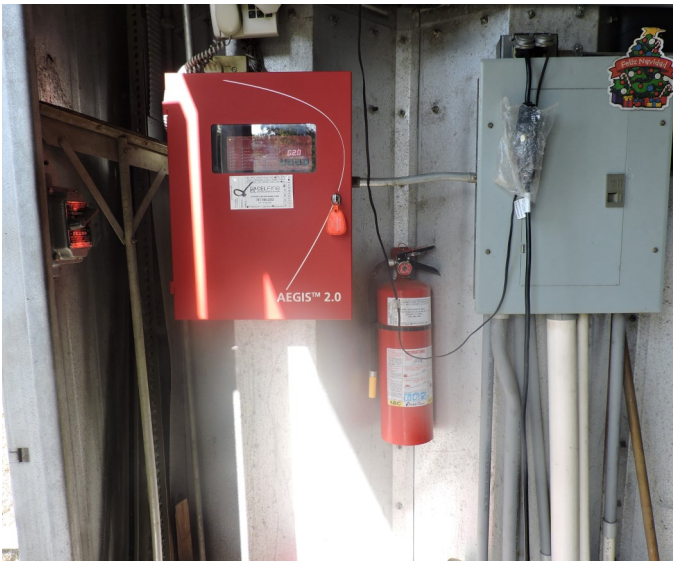
Picture 75 - UPR CENTRAL ACCUMULATION AREA- The room is well vented and provided with ambient controlled temperature in the area and emergency alarm and spill control equipment.
