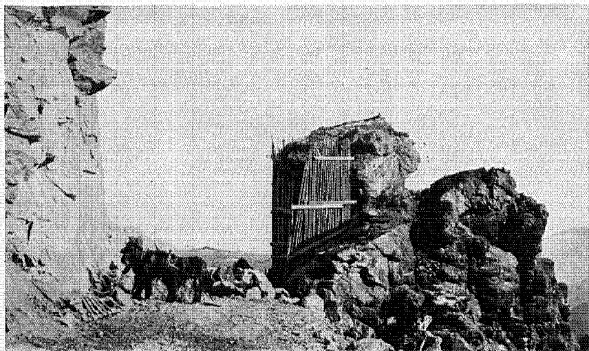
Timber grillages were used to protect scenic cliff formations during the construction period. If all highway builders would follow the same practice, many a beauty spot could be preserved along our public roads
