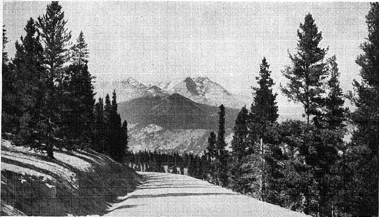
One of the many scenic places along the new Trail Ridge Road. Note the rounded bank to prevent undermining and sloughing
