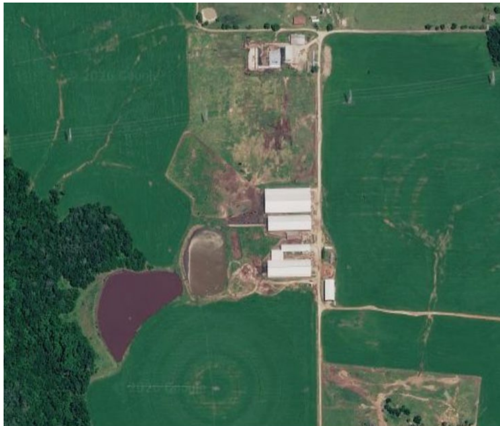
Photo 1: Aerial photo, sourced from Google Earth, depicting the facility and surrounding areas.
