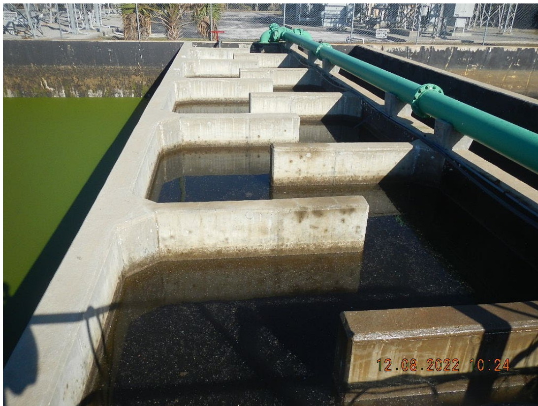
Photo 7. Influent of the Chlorine Contact Chamber. Note small floating particles.
