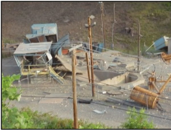
Shaft facility and fan house damaged by an underground mine explosion, Loveridge Mine, Marion County, WV. (Photo courtesy of MSHA.)
