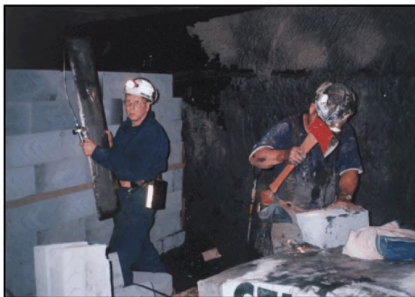
Installing load cells in a ventilation stopping in a longwall headgate to measure load development.
