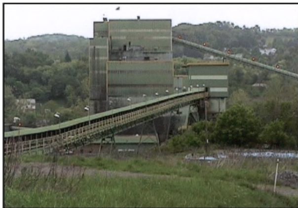
A coal prep plant.
