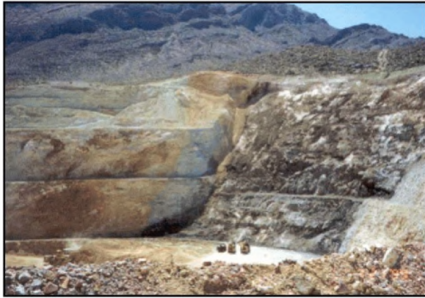
Loose rock, Daisy Mine, Nevada.
