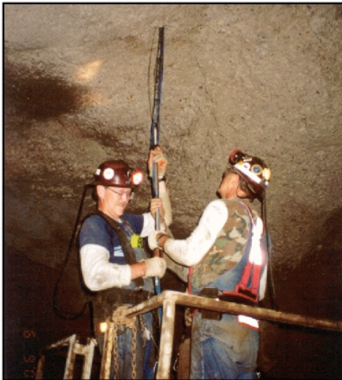
Project personnel install a 40-foot-long vertical borehole extensometer in cemented backfill to monitor displacement during mining beneath the backfill.
