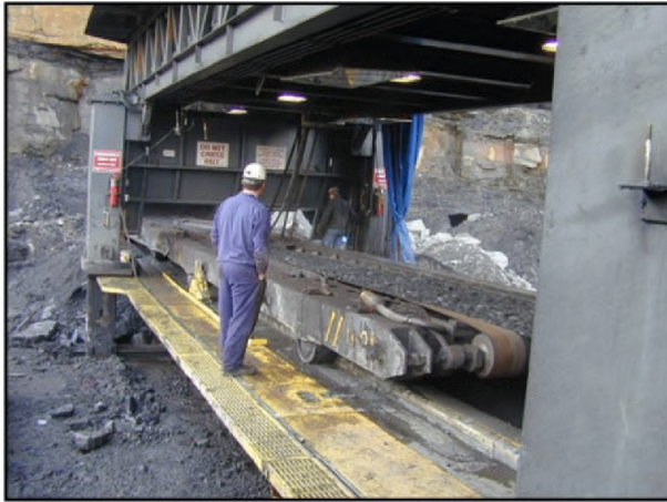
Workers around a highwall mining conveyor system.
