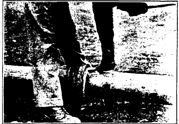
COURTESY U. S. PIPE AND FOUNDRY CO. Calking a lead joint in cast-iron pipe
