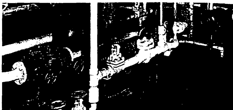
Below—Elliott raw water strainer; driven by two 40-hp, 1200-rpm motors driving hydrogen and lube oil cooling water pumps.
