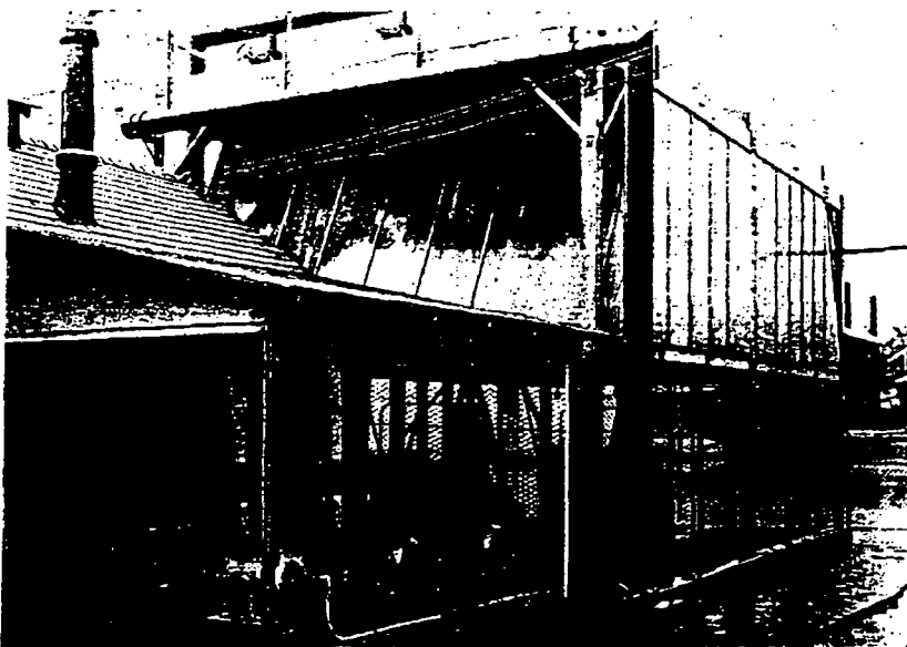
This photograph shows the Fluor-Griscom-Russell Fin-Fan jacket water cooler which serves all four diesel engines. The three circulating pumps shown in the foreground are driven by Elliott Crocker-Wheeler 10-hp, 750-rpm motors.
