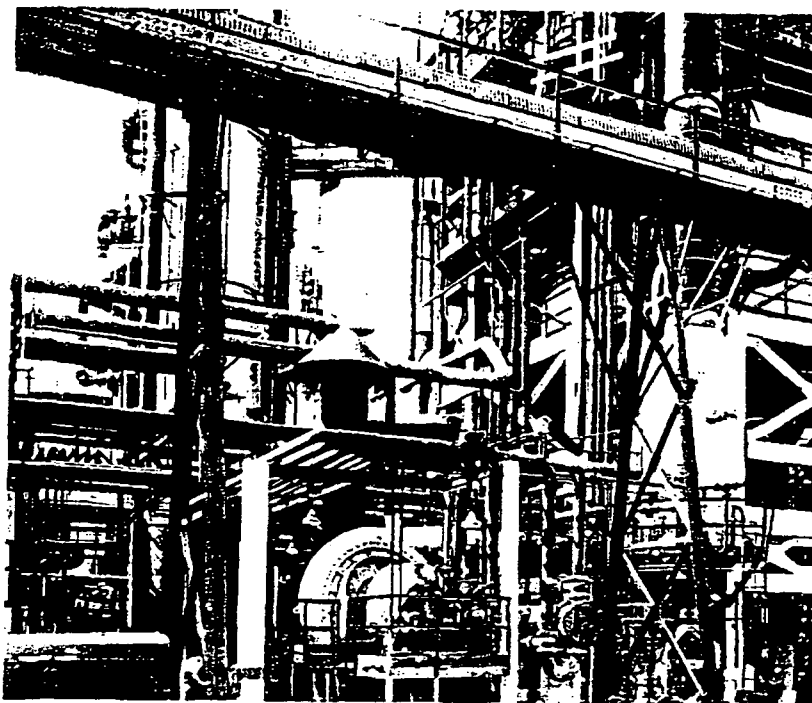
One of the Elliott centrifugal compressors serving a cat cracker. The compressor is rated 52,000 inlet cfm, inlet pressure 14.54 psia, discharge pressure, 35.50 psig, speed 4200 rpm. The 1100-hp turbine takes steam at 350 psig, 436 F and discharges to a condenser at 10 in. Hg abs.
