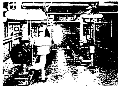
This big ventilating fan is one of four driven by Elliott C-W 20-hp, 1800-rpm motors. Below are station air compressors driven by 75-hp, 1200-rpm motor and two air control compressors driven by 20-hp, 400-rpm motors.
