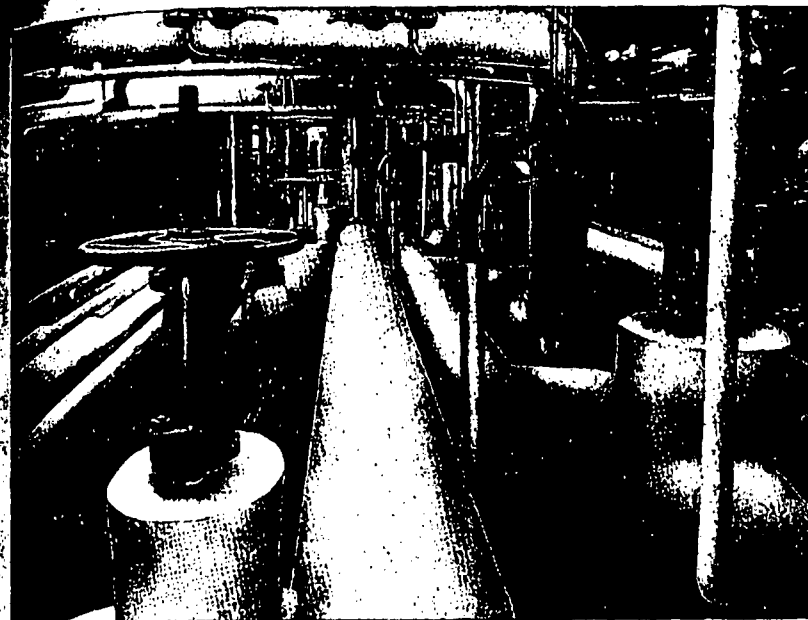
View of Pipe bay in large eastern utility plant, showing pipes insulated with K&M "Featherweight" 85% Magnesia.
