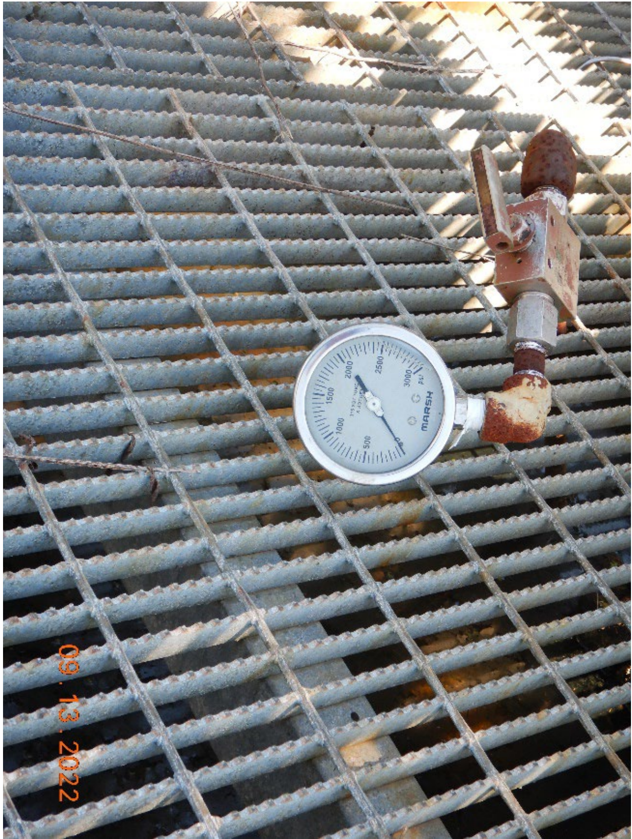
Photograph 3: Looking east, closeup view of surface pressure gauge reading 0 psi.
