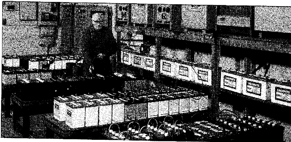
A battery charging facility at a Cape Automotive depot.
