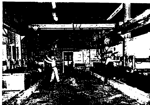
Joe Cantu, electrician 1/c, lowers a large jitney battery in place for a battery charge while Wallace Soulier, electrician 1/c, at right, checks a battery that is ready to come out. There are sufficient space and electrical connections here to charge 36 batteries simultaneously.
