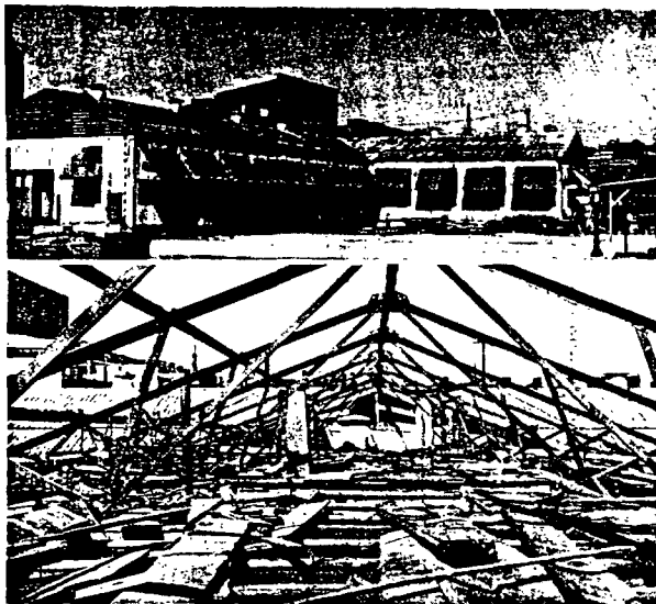
The old Production Planning Building, top photo, finally is torn down after serving as a "temporary" structure for 17 years. In the bottom photo, the partially dismantled building is shown.
