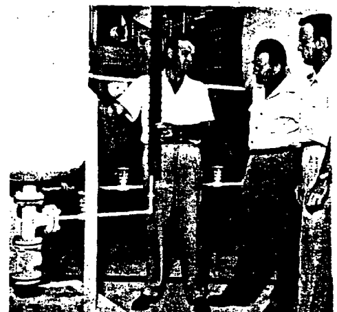
Leo Miller, Frank Padgett, and Burke Grandjean, development engineers, inspect a nitrogen hold-up tank used for the purge gas system feeding into the pilot plant area. It must function according to engineers' specification.
