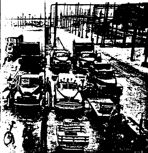
ent types of vehicle are shown in this photo. In back, left to 10-ton crane, 5-ton truck, and "dumpster" truck. Next row: Section pump truck, ton pickup, standard Chevrolet passenger car, road service truck, electric hopper truck, heavy duty fork lift truck, spec scooter, and tractor with trailer. Not nit truck, panel bulldozer.
