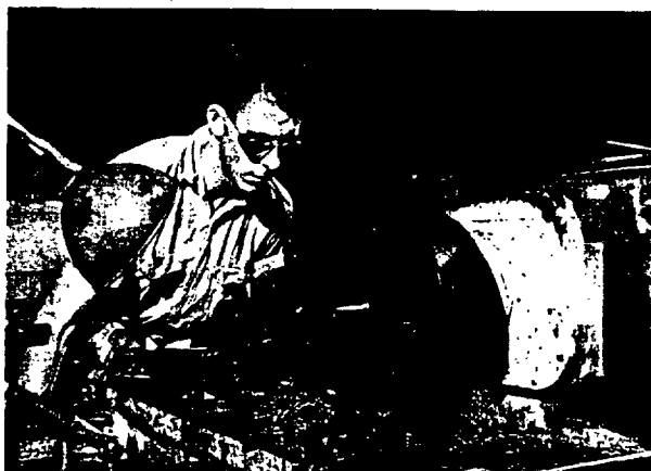
W. J. Landry, inside machinists 1/c, operating a 14-inch lathe, is making an inside thread from a piece of monel stock. The finished product will become a packing gland cap when he is through.
