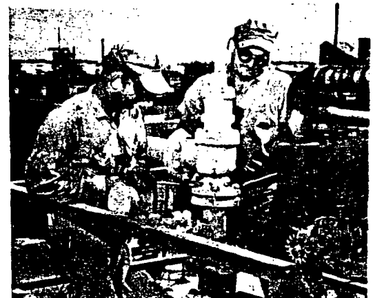
Nolan Keller, left and W. M. Rogillo, mechanical inspectors 1/c, are removing a safety valve for inspection and testing.
