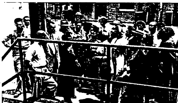
"Rip" Holcombe explains the Compressor House and the Control Room at No. 4 Ethyl Chloride Plant.
