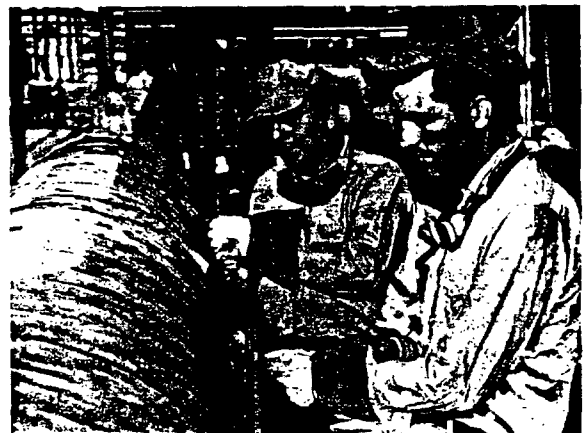
Shown covering a 16-inch line are Sam Fizzillo, insulator 1/c, and A. J. Bourgeois, insulator helper 1/c. Good maintenance on lines such as these prevents steam losses due to rapid condensation.
