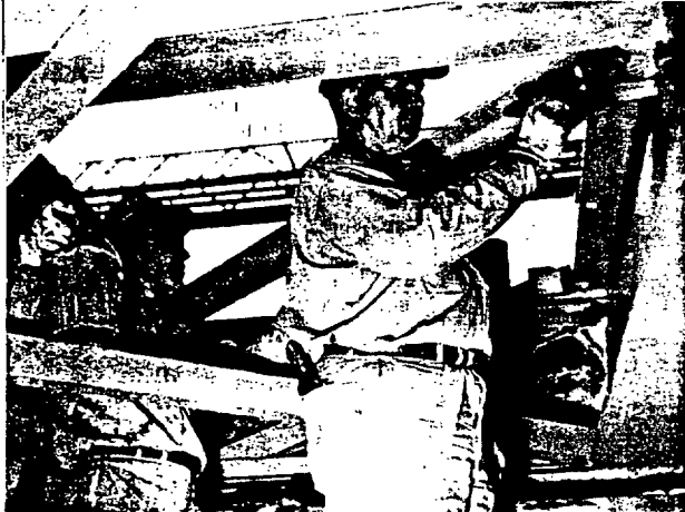
The underside of a railroad support gets a primer coat of paint at the salt dissolving pit. At left is B. T. Bornes, painter helper and Burton Pope, painter 1/c.
