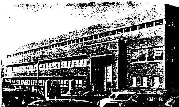
The Medical & Personnel Building, which was completed in 1949, has "grown" considerably in height as a result of the addition of a third story. The addition was completed last month.
