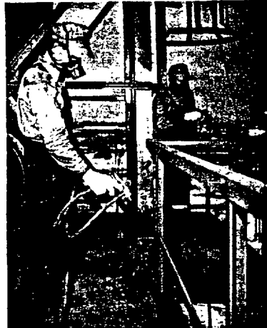
Steeplejack painters Thomas Smith, left, and G. M. Watson spray last coat on chlorine tower in Sodium Area.
