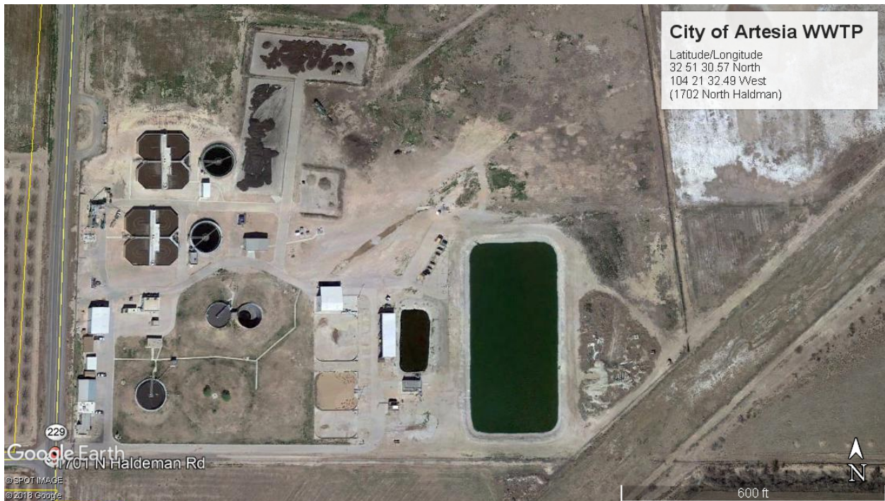
Aerial Image #1: Overall view of the City of Artesia's Wastewater Treatment Plant. Aerial from Google Earth maps.
