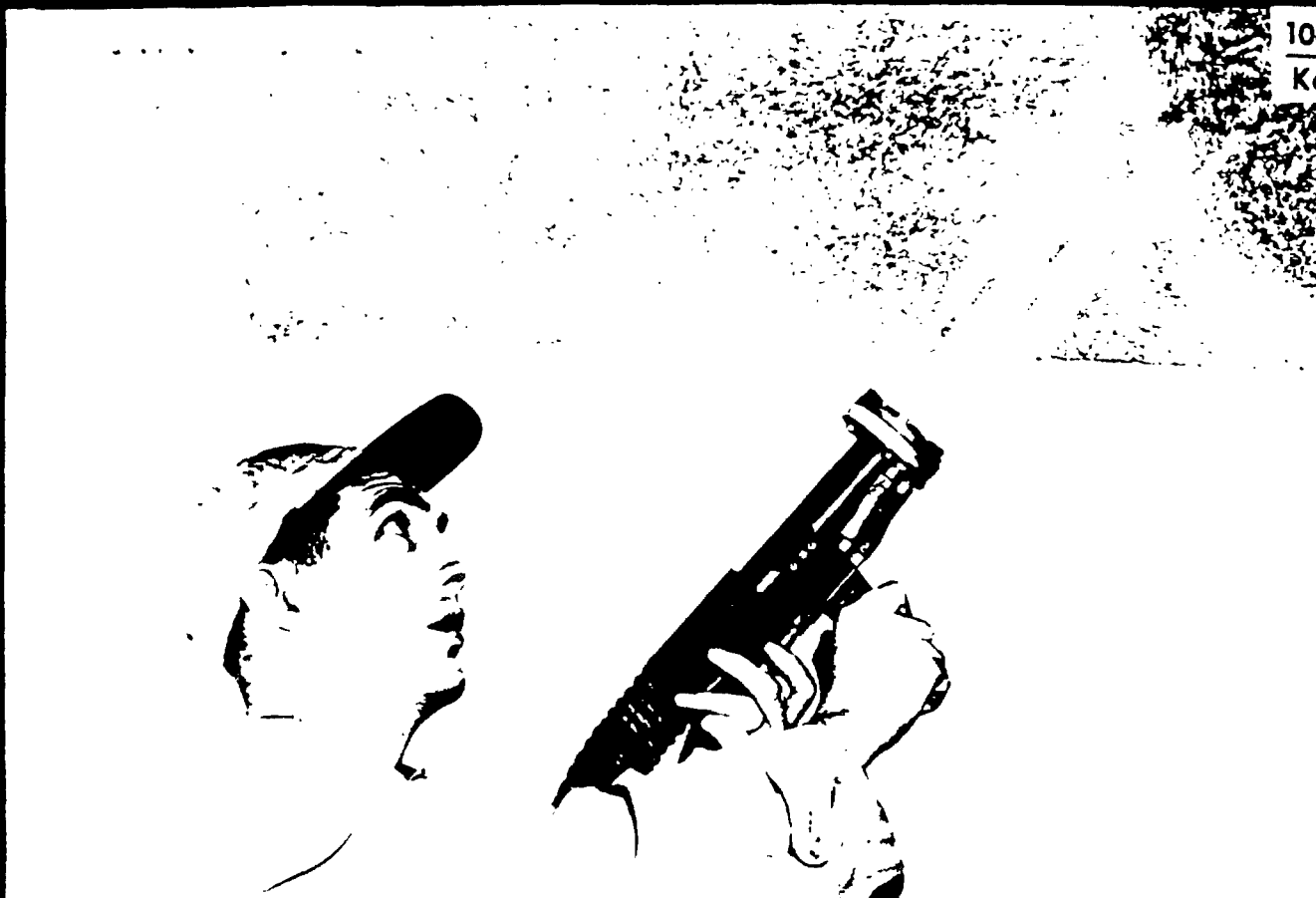
Pure asbestos fibers are "shot" from spray gun in dry state, combine in mid air with misty water spray, and adhere tightly on reaching structural surface.
