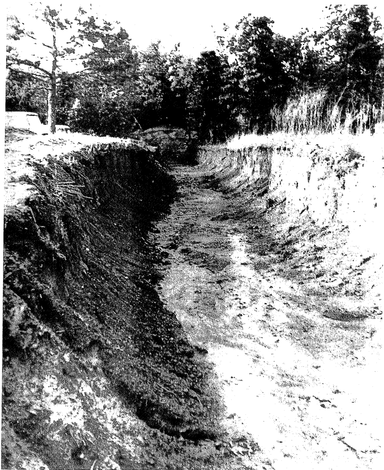
FIGURE 19. - Bulldozer Trench Excavated Prior to Cutting Sampling Trench Clem Vines South Prospect.
