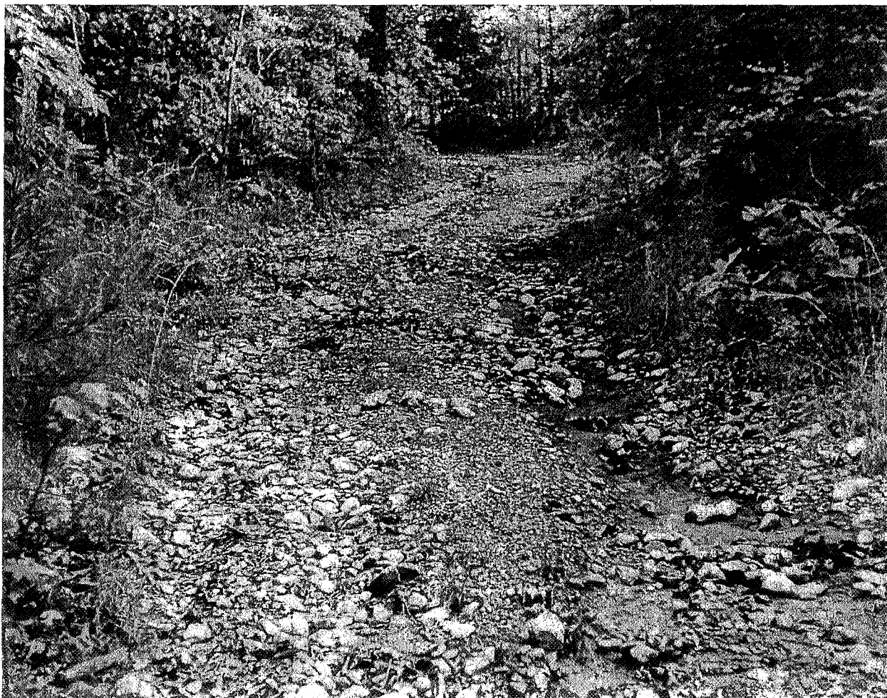
FIGURE 18. - Accumulation of Talc Boulders Along Timber Road.
