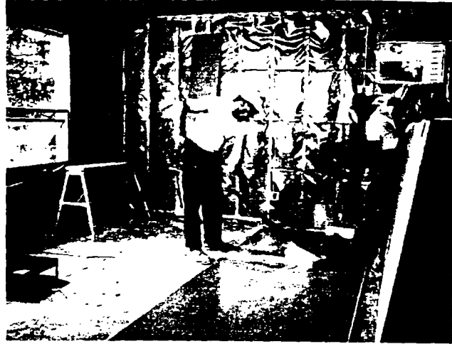
Figure 6-40. Rolling THERMALUX Adhesive Onto Back Of Special THERMALUX Finish Panels
