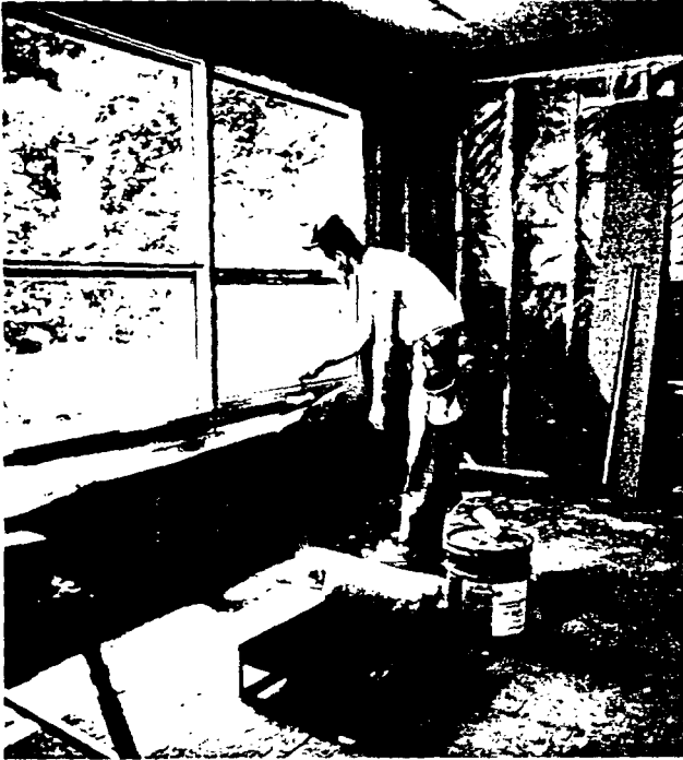
Figure 6-39. Providing For Plenty Of Ventilation Before Working With THERMALUX Adhesive or THERMALUX Solvent
