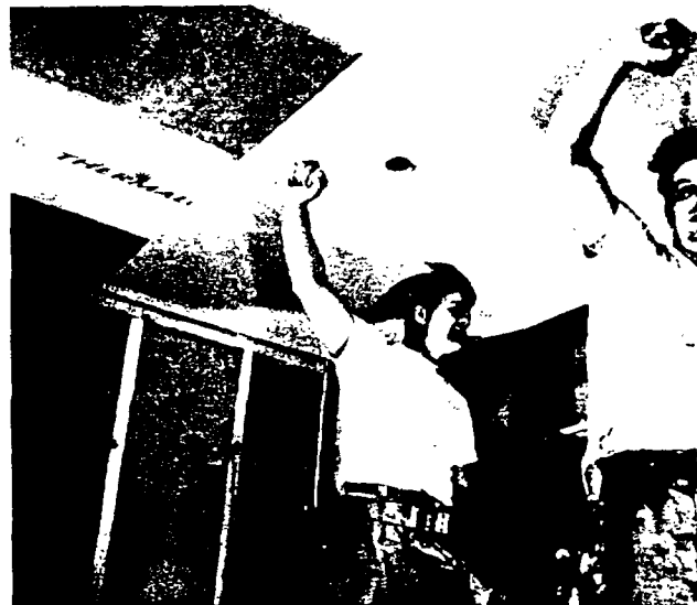
Figure 6-44. Smoothing Panel Into Preliminary Lamination
