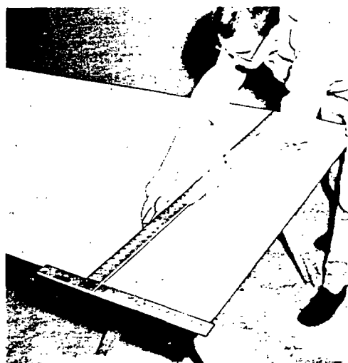
Figure 6-15. Cutting Heating Panel by Scoring through Electrodes and Heating Element
