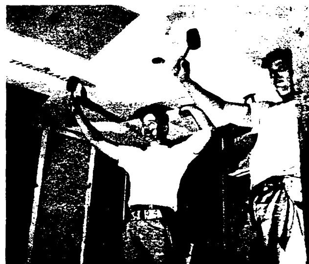
Figure 6-45. Impacting Face Panels For Positive Lamination
