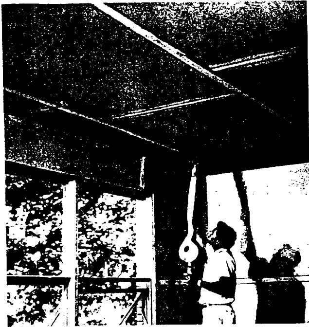
Figure 6-48. Joint Taping Finish Panel In Normal Manner With Materials Recommended
