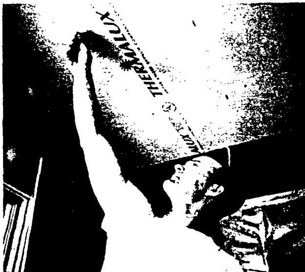
Figure 6-42. Testing dryness of adhesive to be certain it is sticky, but not wet, when finish panels are adhered. Similar test on adhesive-coated finish panels governs time that lamination takes place.
