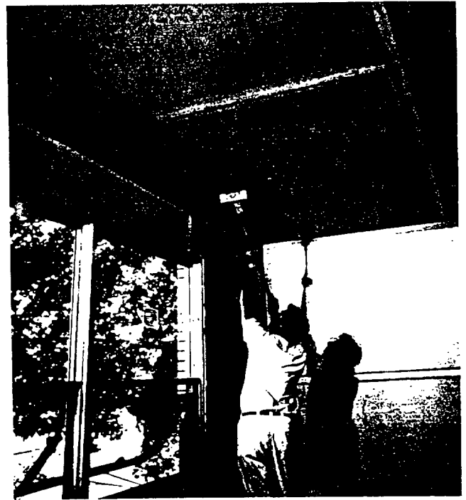
Figure 6-50. Topping Joint In Finish Panel
