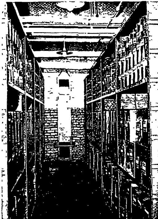
FIG 34-13 - A well designed flammable liquid storage room with both high and low level ventilation and automatic fire extinguishment. Ventilators are designed for 12 air changes per hour
