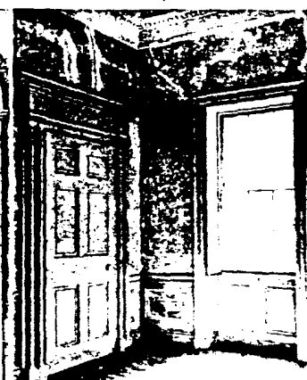
Woodwork first coated, walls in preparation for white lead paint
