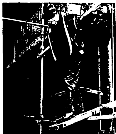
Safety Engineer Bob Palmer shows how a "near miss", that could have been a fatal fall, happened. When an employee stepped on an untied board of a scaffold, it "kicked up" and caused him to fall about five feet. Luckily, the employee was unhurt. However, he fell within about two feet of a roof edge and a 40-foot fall.
