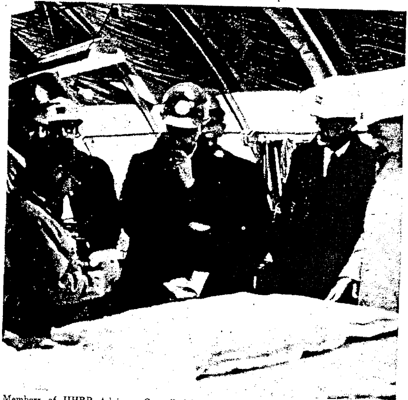
Members of IIHRP Advisory Council joined hygienist team in visit to Oyster Creek generating station construction site in Toms River, N. J. Observing a sawing operation are Drs. Selikoff, Hammond and Pundsack.
