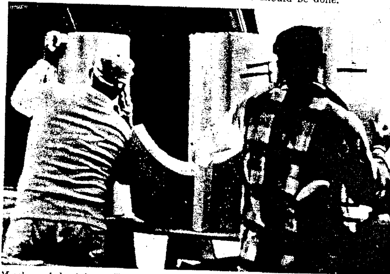
Members of the Asbestos Workers Union install pipe covering in Oyster Creek generating station now being built at Toms River, N. J. Site was visited by IHRP team. (See story on page 8)
