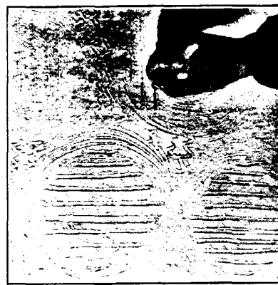
This novel finish is accomplished by means of a wad of cloth and a blunt stick or other tool
