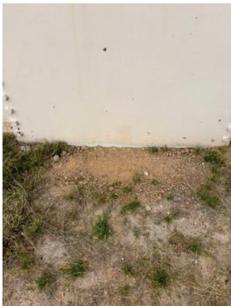
Vol Andia Storage Tank # 02 (hole filled and packed)
