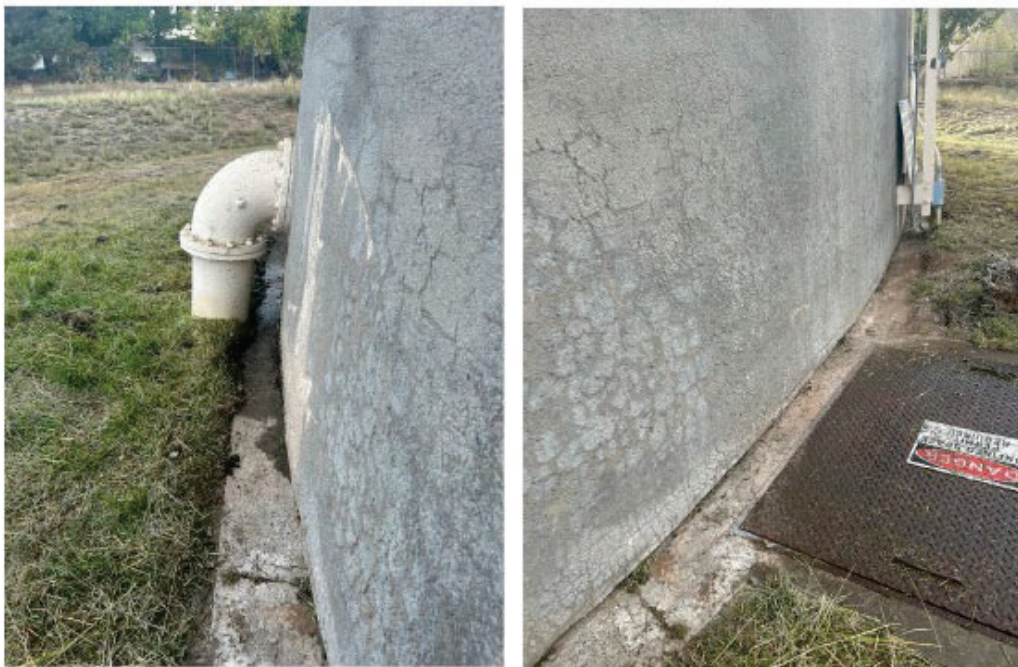
Glennwood Storage Tank (vegetation removed)
