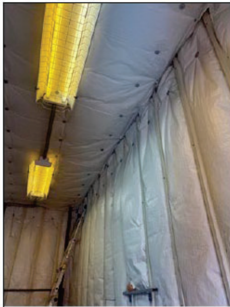
Burton #1 Treatment Unit (insulation repair)
