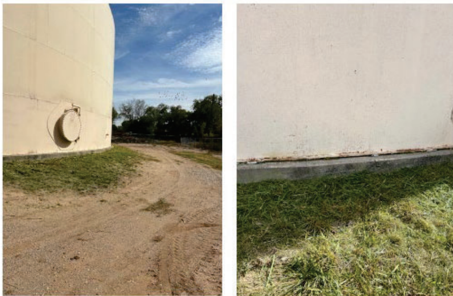
Griegos Storage Tank (vegetation removed)
