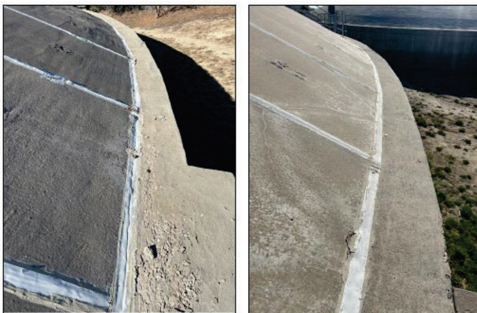
Lomas Storage Tank #02 (vegetation removed)
