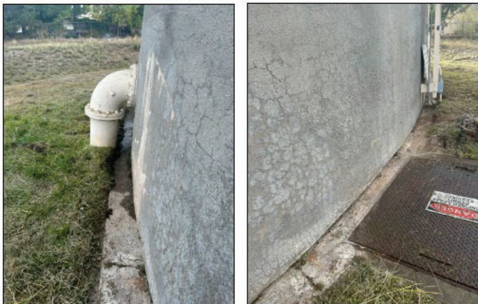
Glennwood Storage Tank (vegetation removed)
