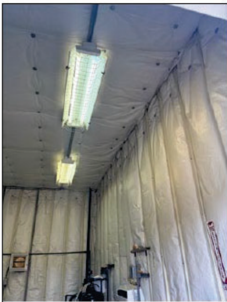
Burton #1 Treatment Unit (insulation repair)
