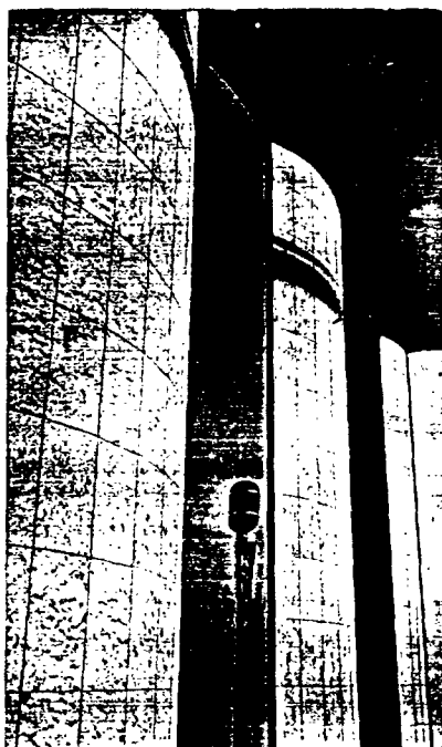
In Station KSL, Salt Lake City, ACOUSTONE tile on curved wall panels control reverberation and give studio performances new clarity and brilliance.
