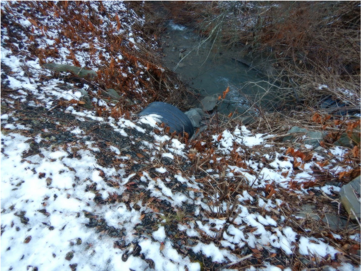
DSCN4066 Meredith Creek Culvert (approximately 100 ft east downslope of driveway)
