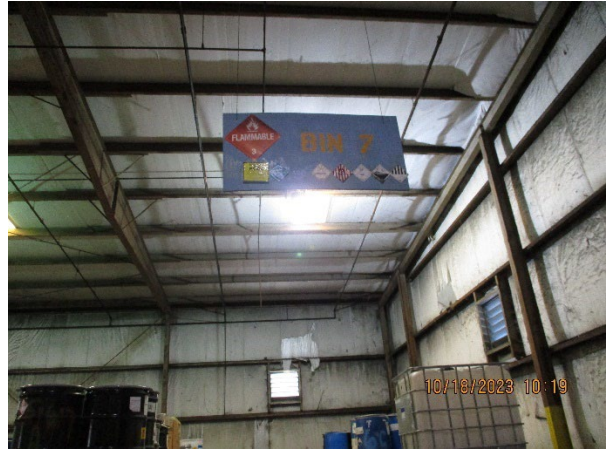
Photo 10: Building 2 Container Storage Areas
