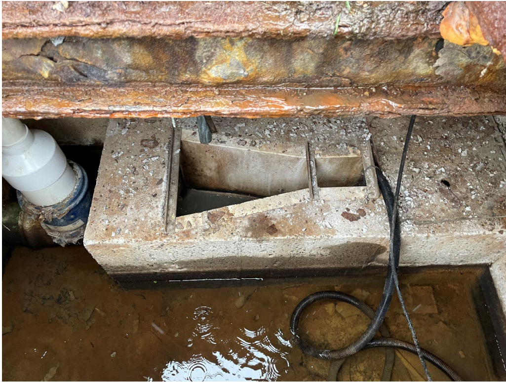
Photo #3. The Parshall flume w/ the flow sensor is recording high flow due to turbulence.
