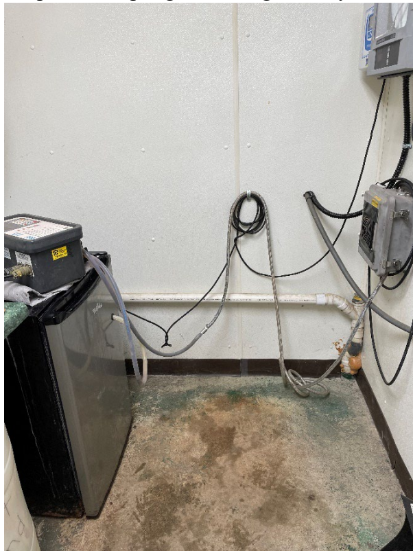
Photo #2. The facility's composite sampling assemblage is dirty and/or contains algal growth.
