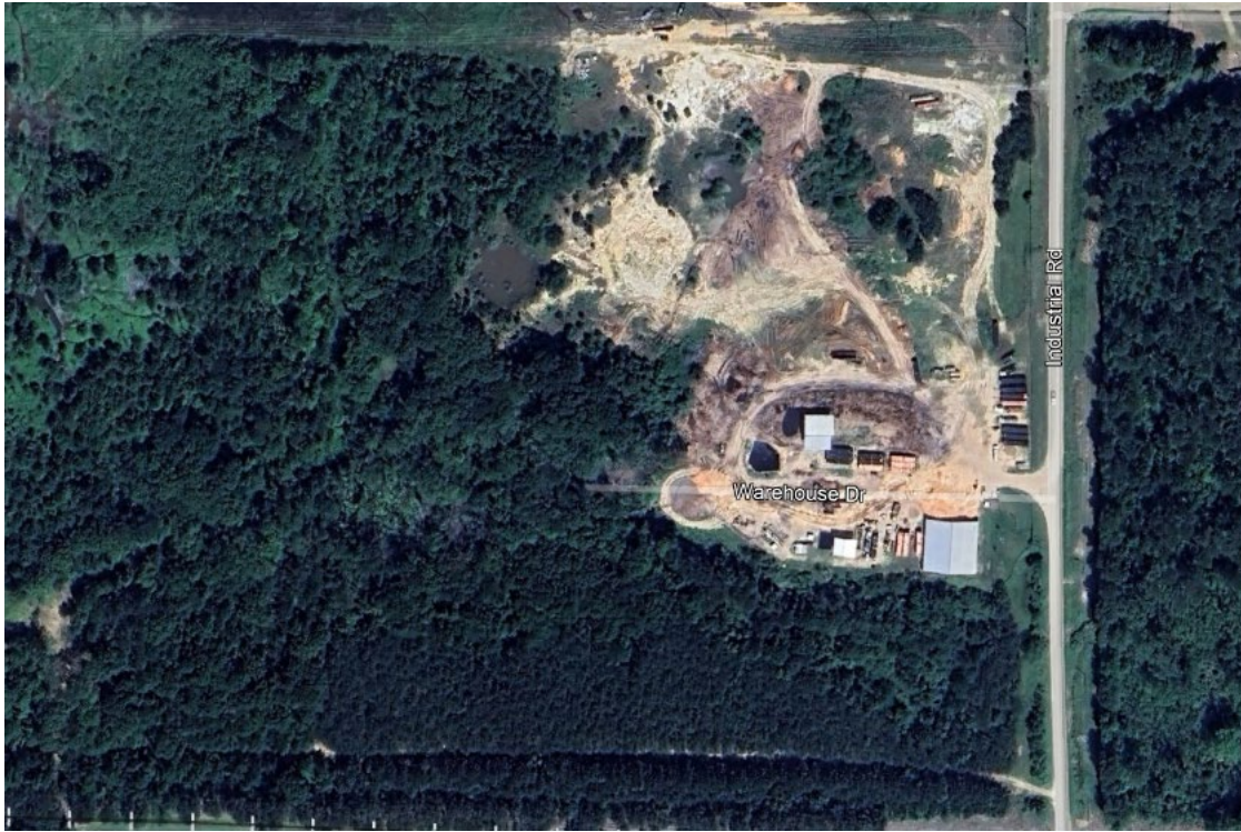
Aerial Image 1. Overview of USA Disposal facility. Google Earth image date 05/14/2023.
