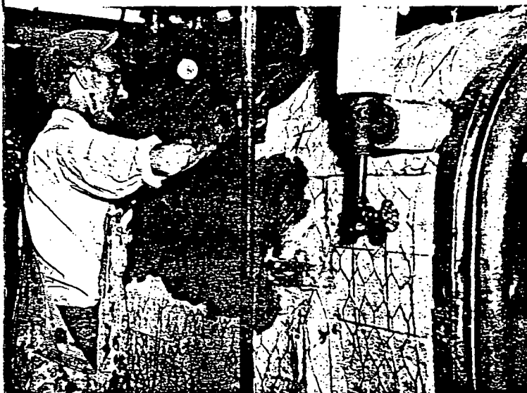
41. Asbestos cement being applied over hexagonal mesh on block insulation
