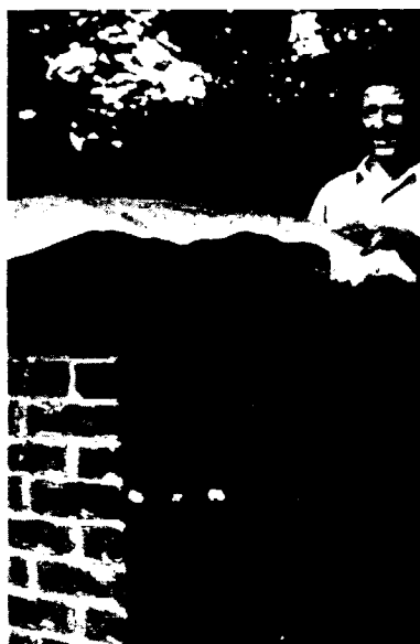
Views showing rebuilt chimney, without lead cap, dressing the lead over the chimney cap, and the finished lead chimney cap in place, adequate protection against deterioration
