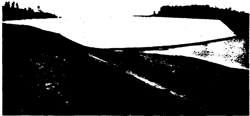
Full view of the steel-faced South Catamount Creek Dam, Colorado Springs, Colo., the exposed face primed with red lead and finished with pure white lead and oil paint
