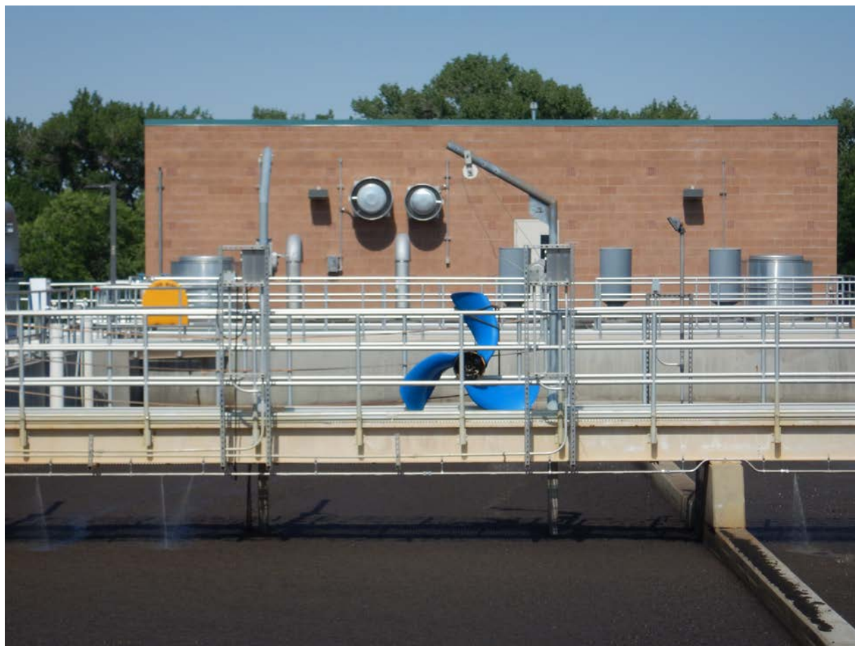
View of removed "banana blade" from one (1) of the Medium Rate Activated Sludge (MRAS) basins. July 10, 2018 10:15 AM (DSCN0879).
