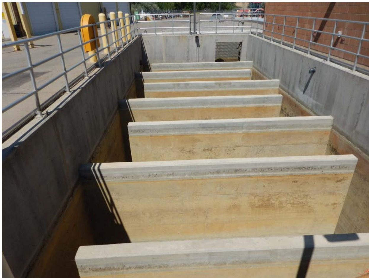
View of the previously used Chlorine Contact Basin 1 in the disinfection process. July10, 2018 11:16 AM (DSCN0901).
