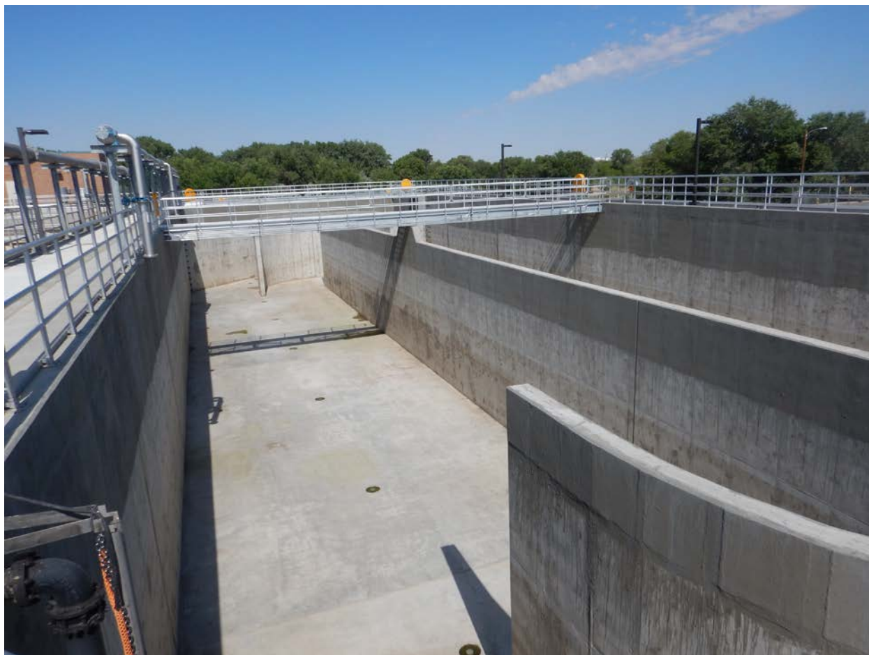
View of the newly constructed third MRAS structure awaiting equipment installation (diffusers). July 10, 2018 10:17 AM (DSCN0880).
