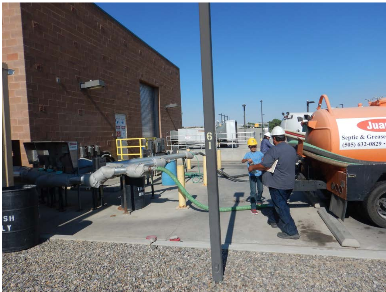
View of the City of Farmington's septage receiving location at the entrance of the WWTP. July 10, 2018 9:15 AM (DSCN0855).
