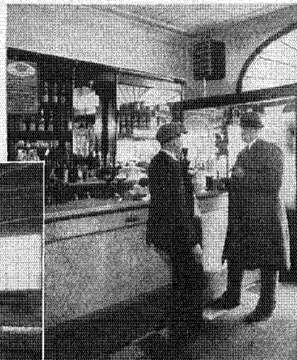
Here are three typical installations of Venturafin Heaters—a factory, an airplane hangar and a small drug store. Originally these units were designed to heat large spaces in factories, but now they are being used in garages, gas-filling stations and even in some private homes. Note that the units and piping are placed overhead, out of the way
