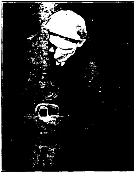
(LEFT) Joint ready to pour, with collar and clay gate in place.
