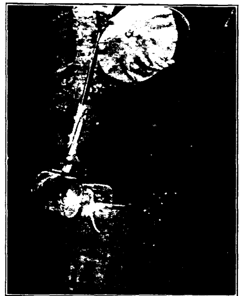
(LEFT) Joint ready to pour, with collar and clay gate in place.
