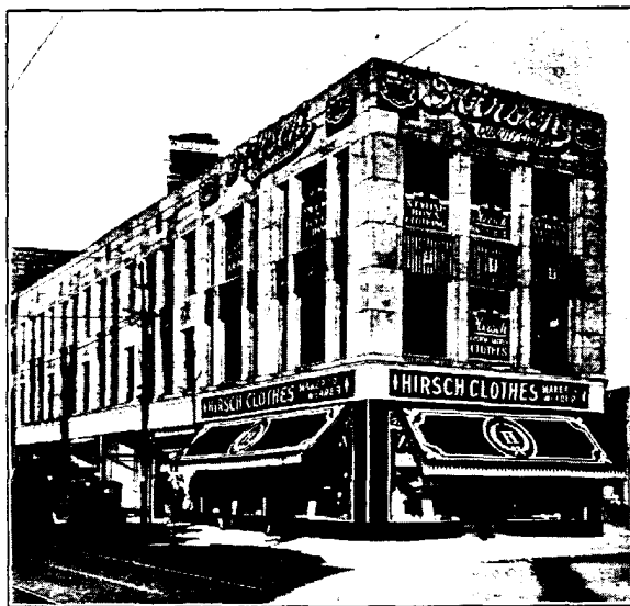
A Chicago building in which macotta lead spandrels have been used.
