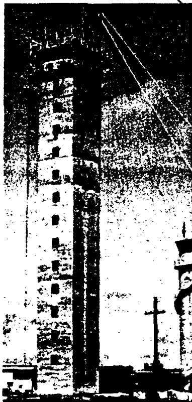
The 166 foot high control tower on Guam, in the construction of which Vinnell introduced the use of slip formed walls of concrete.
