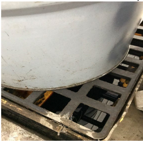
Photo-13 CAA- Used Oil in Secondary Containment
