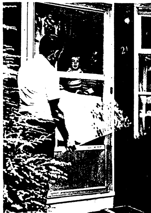
Storm window replacement and patio doors are growing safety glazing applications for shatter-resistant Acrylite cast acrylic sheet.
