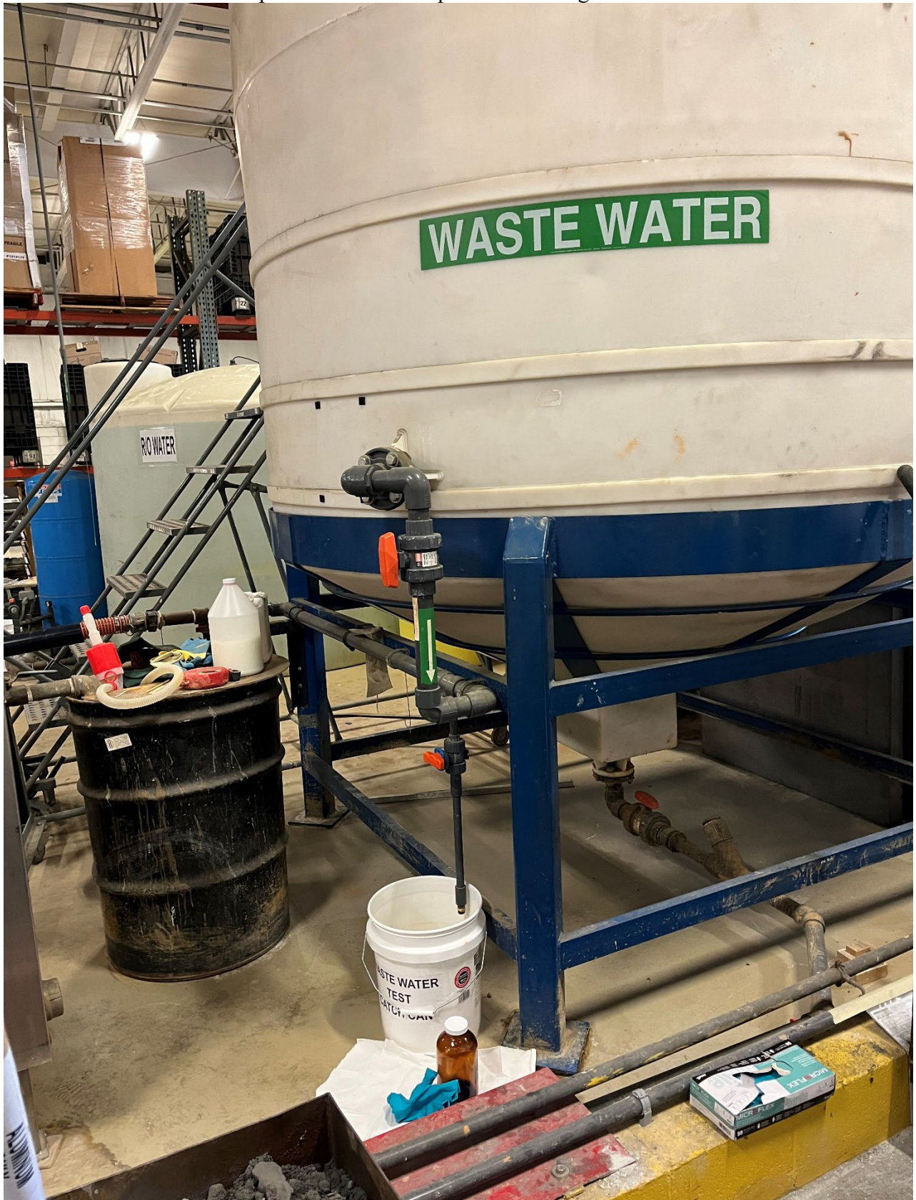
Photo #1: View of the sample location for the process discharge to the local POTW.
