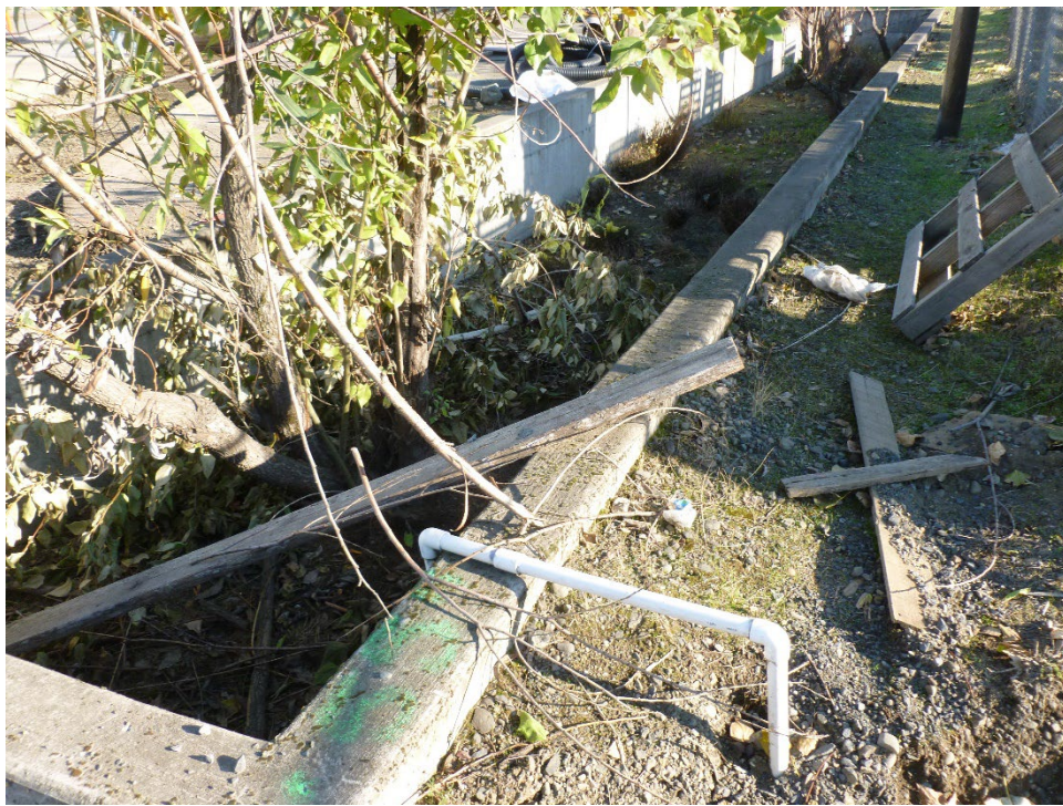
Photo 5/P1010536 – Infiltration Planter
