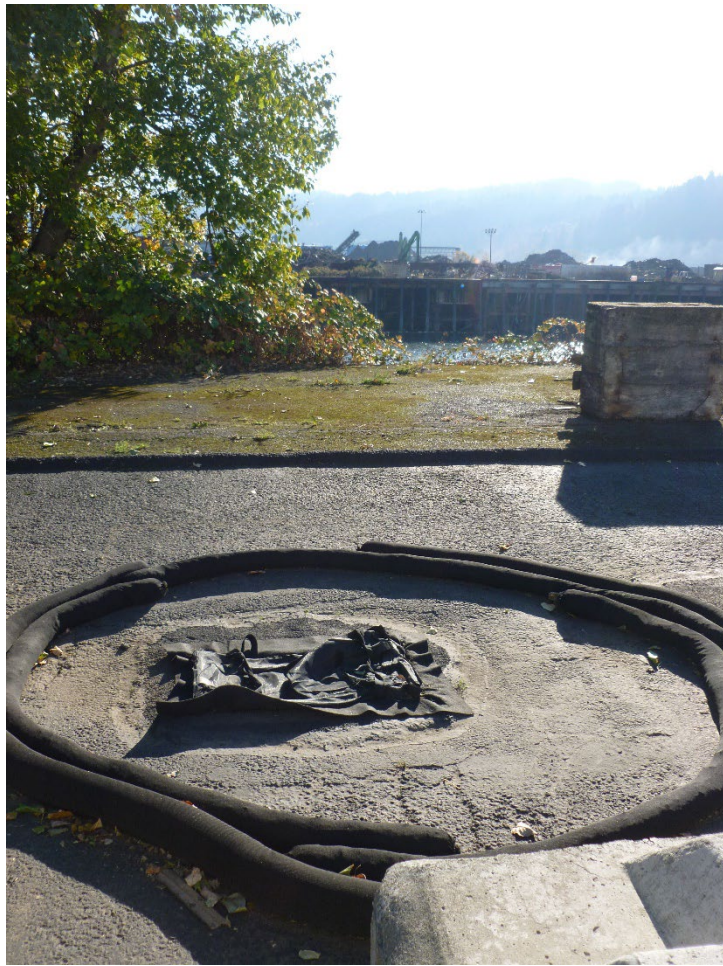
Photo 3/P1010530 – Catch Basin 4
