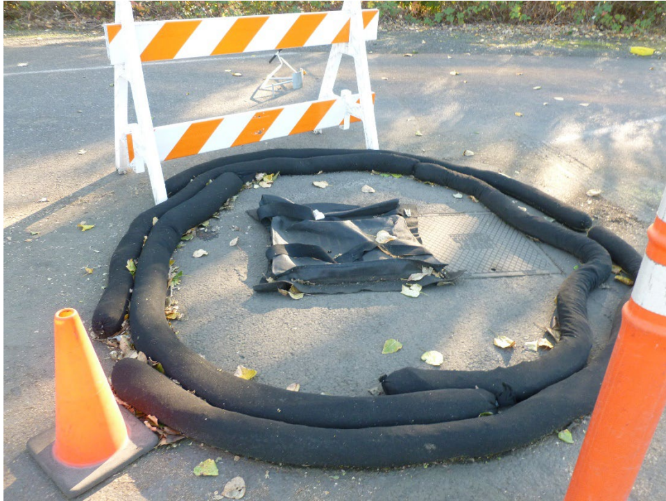
Photo 1/P1010537 – Catch Basin 1
