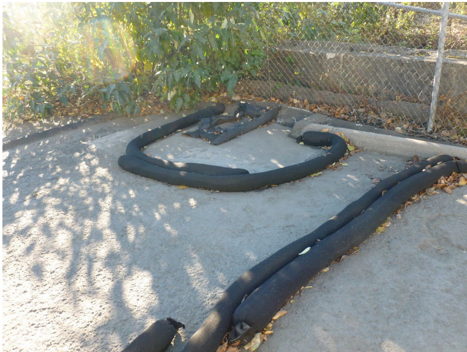
Photo 2/P1010532 – Catch Basin 2
