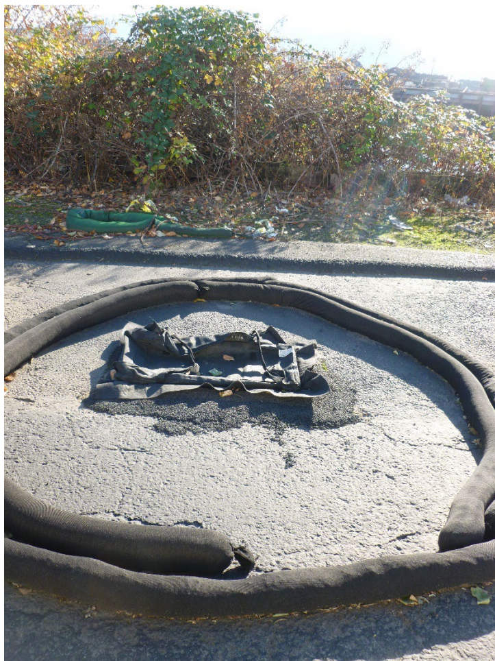
Photo 4/P1010531 – Catch Basin 5
