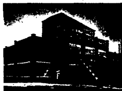
Union Iron Works
