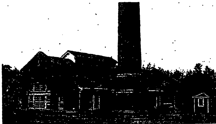
The power house at Willmar.
