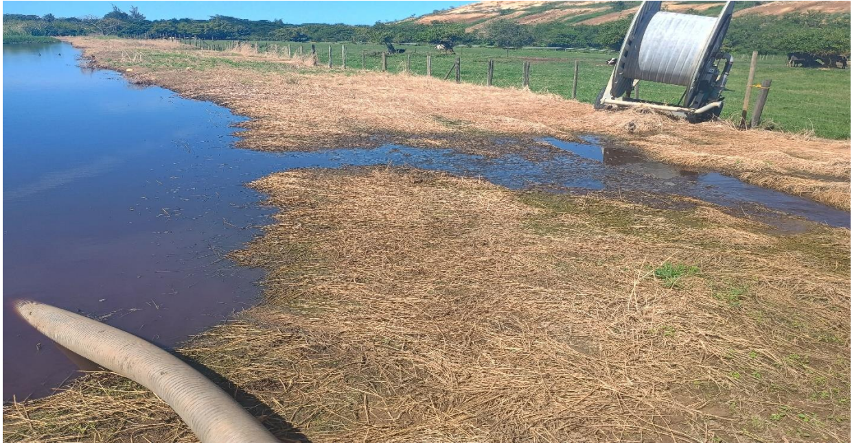
Depicts a view of the liquid manure storage lagoon with no freeboard and overflowing towards the pasture. The overflow was located at the northeast side corner of the lagoon.
