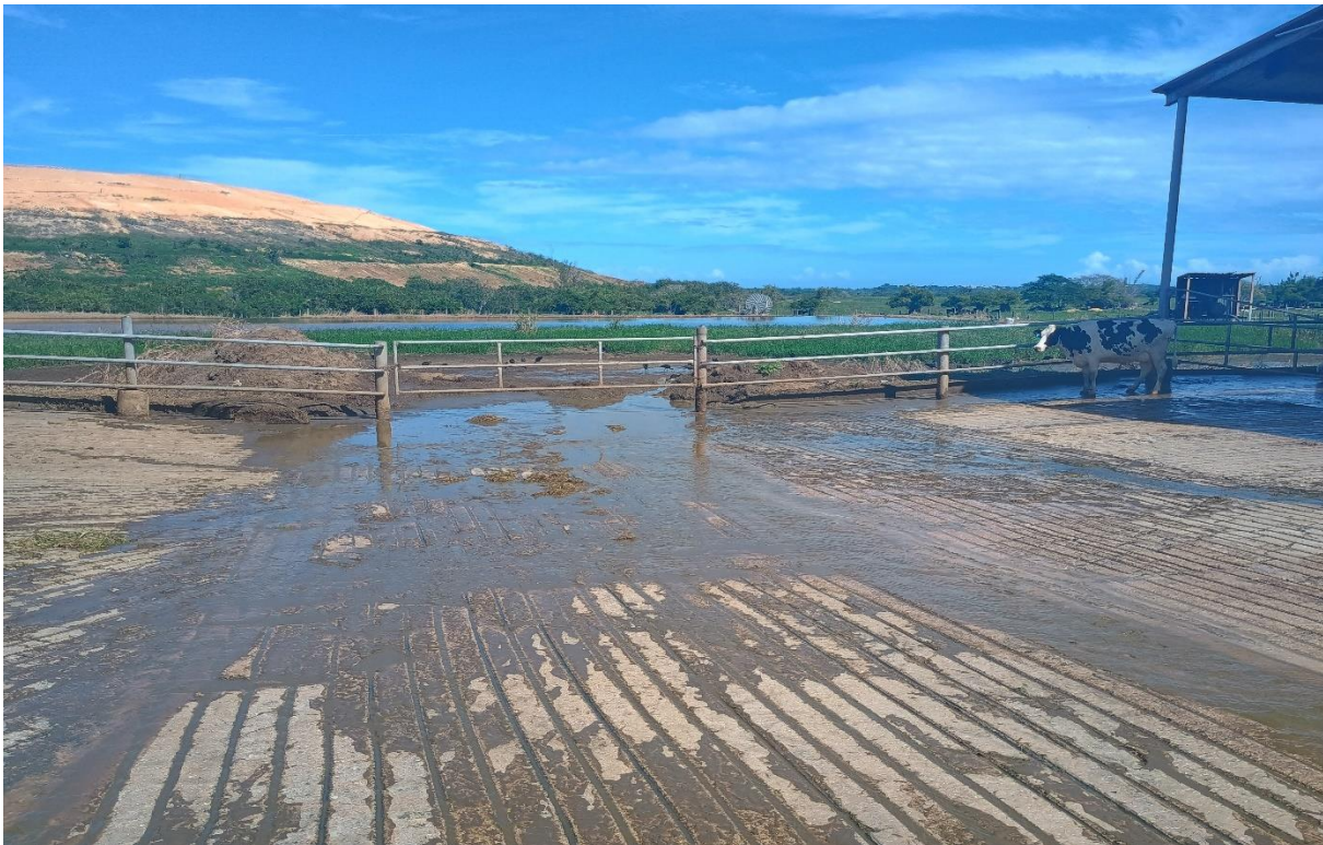
Depicts a view of the manure that comes from the feeding barns drainage area that flows via gravity into the manure storage lagoons.
