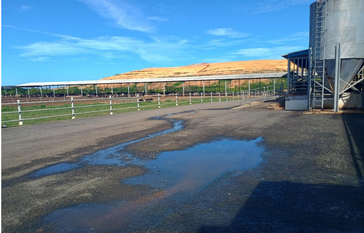
Depicts a view of the dairy farm facility entrance. Stormwater runoff from adjacent field pasture was observed in the pavement.
