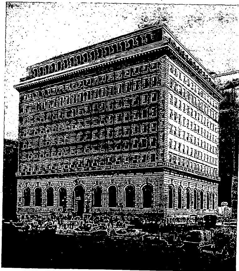
Federal Reserve Bank of Cleveland
