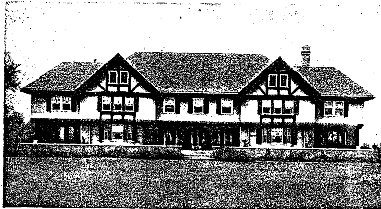
Fig. 4. House at Hinsdale, Ill. Brown Stain Used in Connection with Grey Plaster Is Usually Pleasing
