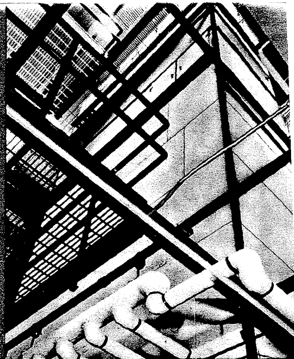
Coating tower, 41 feet high, built and insulated with Johns-Manvil Marinite by Electro Technical Products, Nutley, New Jersey.
