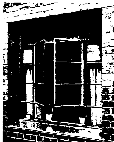
Detail of window sash sill and lintel with fresh coat of rust inhibiting red lead paint.
