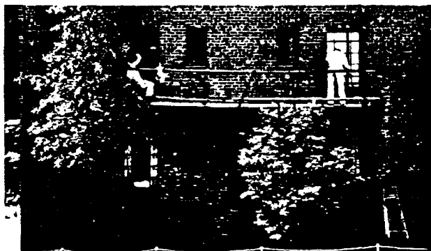
Detail of window sash sill and lintel with fresh coat of rust inhibiting red lead paint.
