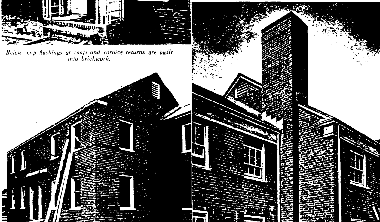
Completed flashings to walls and chimney and at cornice returns.
