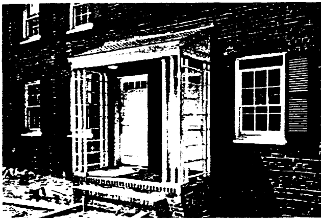
Completed porch showing flashings in place.
