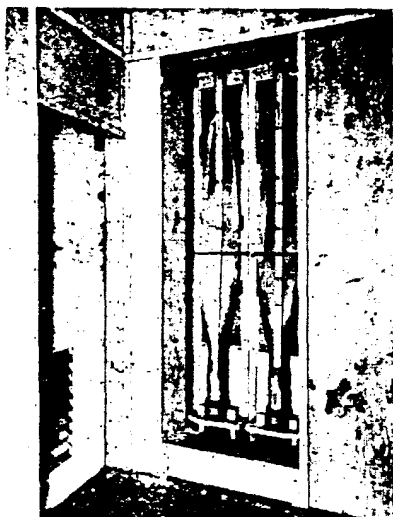
Blades in exposure position in X-ray room. Note walls constructed of laminated lead-plywood panels secured with lead head nails.
