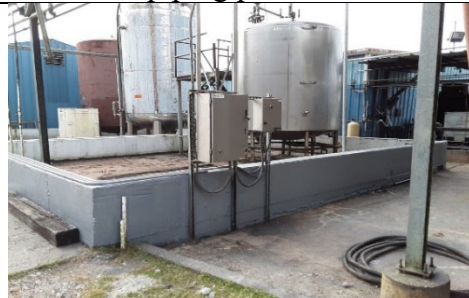
Photo-15 Production Area #4, painted Diked Walls
