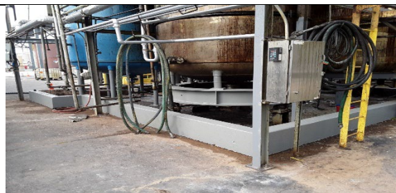
Photo-13 Production Area #3, Chipped diked wall repainted
